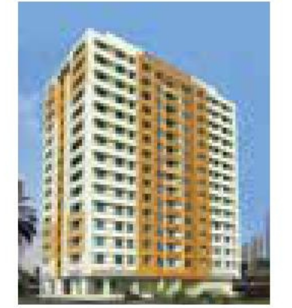
FRANKFURT SPORTS TOWER 1 HANDLED OVER
